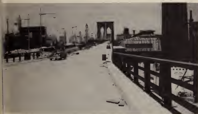
The repaved roadway of the Brooklyn approach, Manhattan-bound. Chimney stack is part of the old power house for cable-car operation which started in 1883. The building in recent years has been used as a Department of Public Works Shop, which is scheduled to be torn down in the near future.
